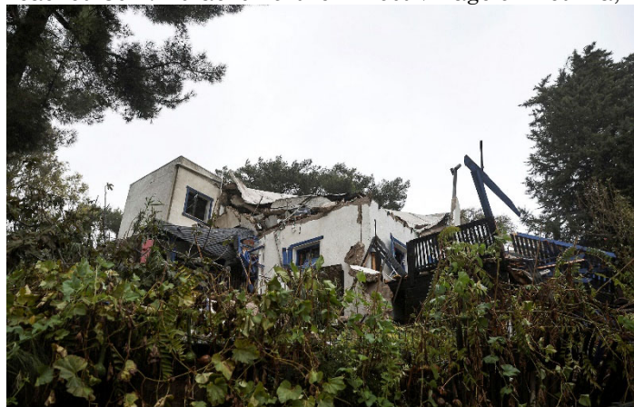
A house damaged by Hezbollah in Kibbutz Manara on November 27, 2023 (AFP)
